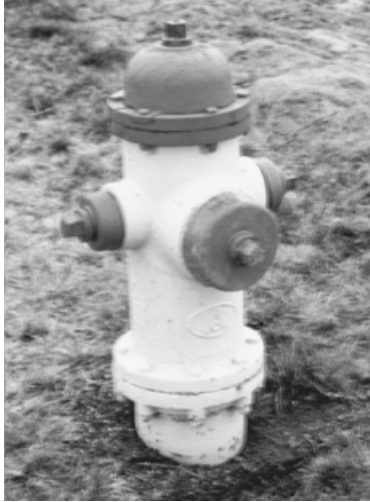
FIGURE 6.75 Dry barrel hydrant.
