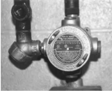
FIGURE 5.29 Explosion-proof junction box.
