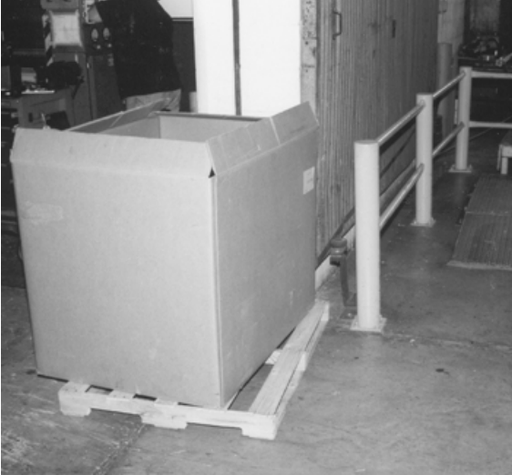
FIGURE 6.8 Blocked fire door.
