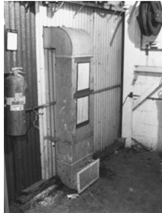
FIGURE 5.26 Floor level ventilation.
