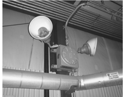
FIGURE 4.13 Emergency lights for a hazardous location.
