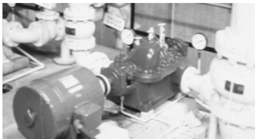
FIGURE 6.71 Fire pump, electric, horizontal shaft.
