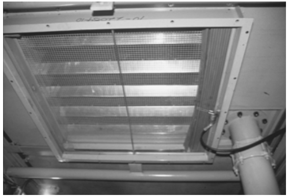
FIGURE 6.86 Carbon dioxide system vent closer.
