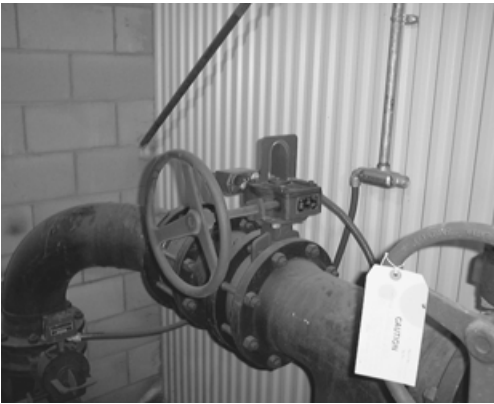
FIGURE 6.55 Butterfly valve.
