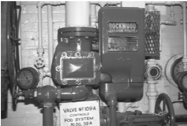
FIGURE 6.46 Deluge sprinkler valve.
