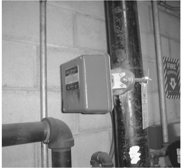
FIGURE 6.39 Flow switch.
