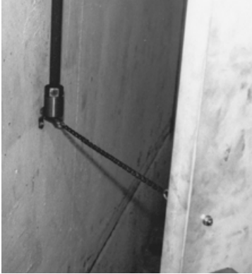
FIGURE 6.85 Carbon dioxide system door closer.
