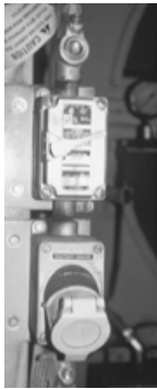
FIGURE 5.31 Explosion-proof outlet.
