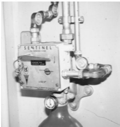
FIGURE 6.98 Dry chemical system.
