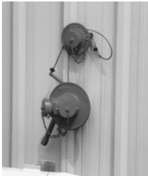
FIGURE 6.77 Wall hydrant.
