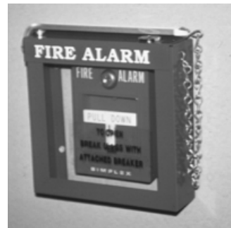
FIGURE 6.10 Pull station with tamper-resistant cover.
