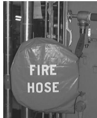
FIGURE 6.24 Standpipe hose station, class I.
