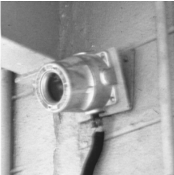
FIGURE 6.19 Flame detector.
