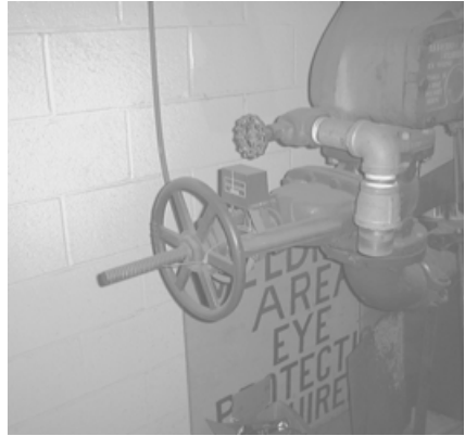
FIGURE 6.54 Outside screw and yoke (OS & Y) valve.
