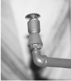
FIGURE 6.59 Air aspirating foam sprinkler head.
