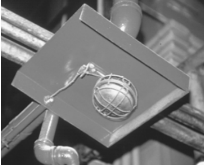
FIGURE 6.17 Heat detector, HAD type.
