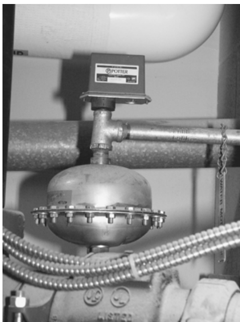
FIGURE 6.38 Pressure switch.
