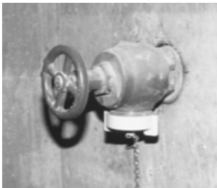
FIGURE 6.24 Standpipe hose station, class I.
