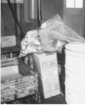
FIGURE 7.49 Obstructed access to extinguisher.
