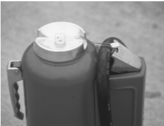
FIGURE 7.9 Top of cartridge operated dry chemical extinguisher.
