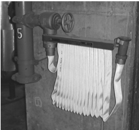
FIGURE 6.26 Standpipe hose station, class III.
